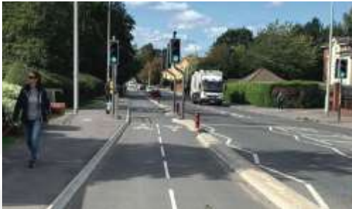
Two way segregated cycleway.
