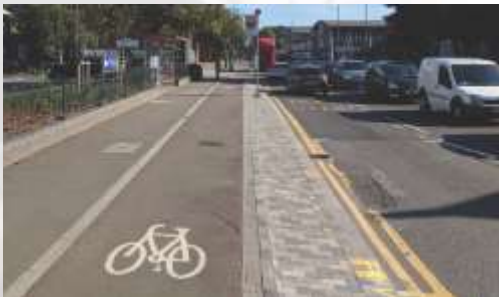
On road segregated (stepped) cycleway.
