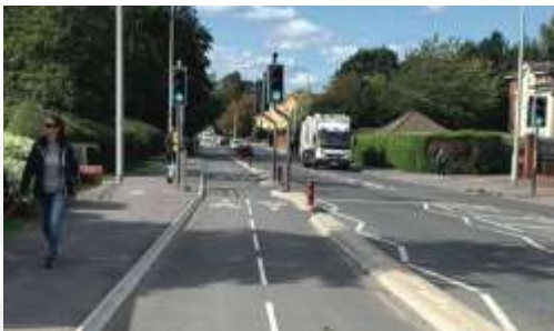
Two way segregated cycleway.
