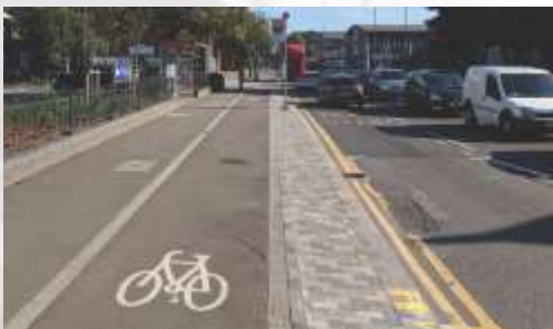
On road segregated (stepped) cycleway.
