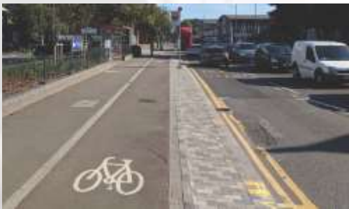
On road segregated (stepped) cycleway.
