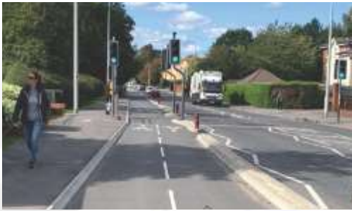
Two way segregated cycleway.
