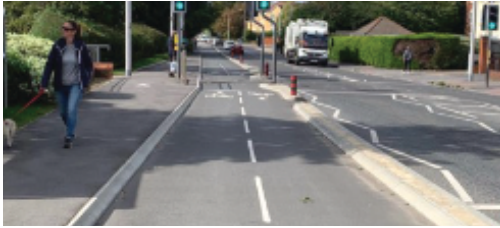
Two way segregated cycleway.
