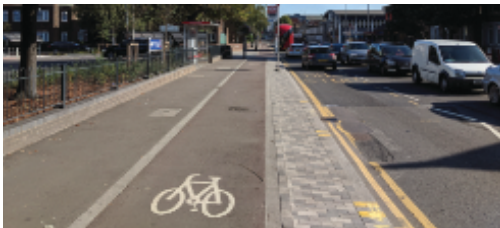
On road segregated (stepped) cycleway.
