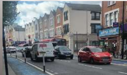
Lightly segregated cycleway.
