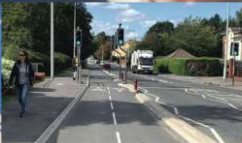
Two way segregated cycleway.
