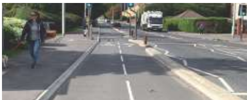
Two way segregated cycleway.
