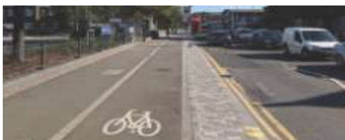
On road segregated (stepped) cycleway.
