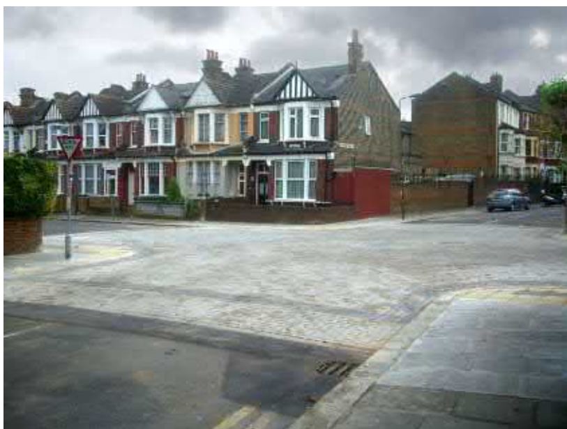
Figure 4.9. Raised table junction
