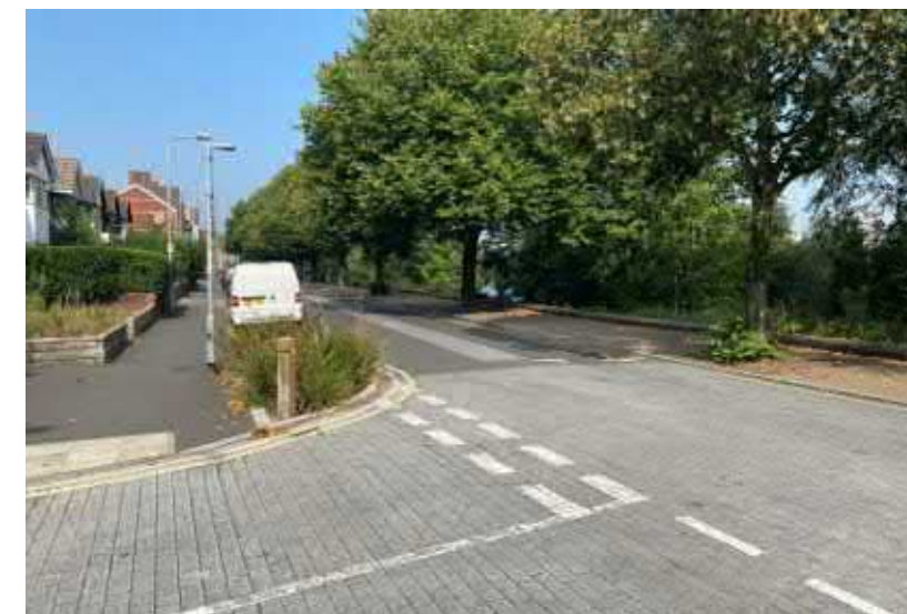
Figure 4.7. Buildouts with SUDs
