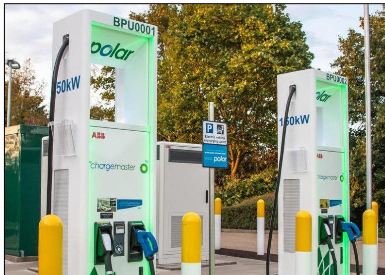
150kW electric vehicle chargers of the type that could be used to charge the new ferry
