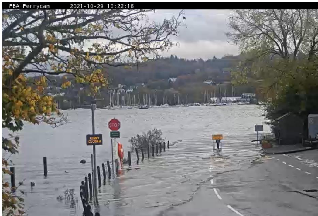
The Ferry House (west) slipway with the lake water level at 2.1m (from Ref. N)
