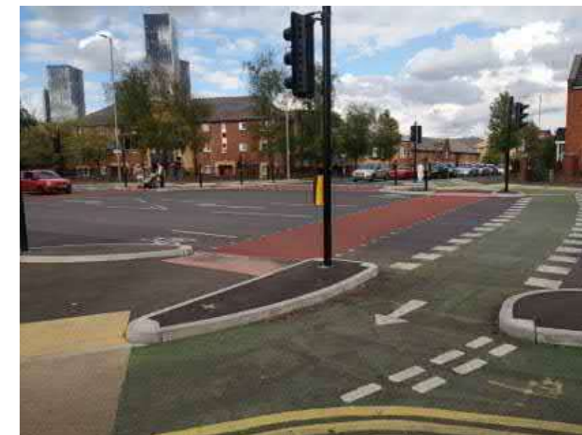
Figure 3.13. CYCLOPS signalised junction
