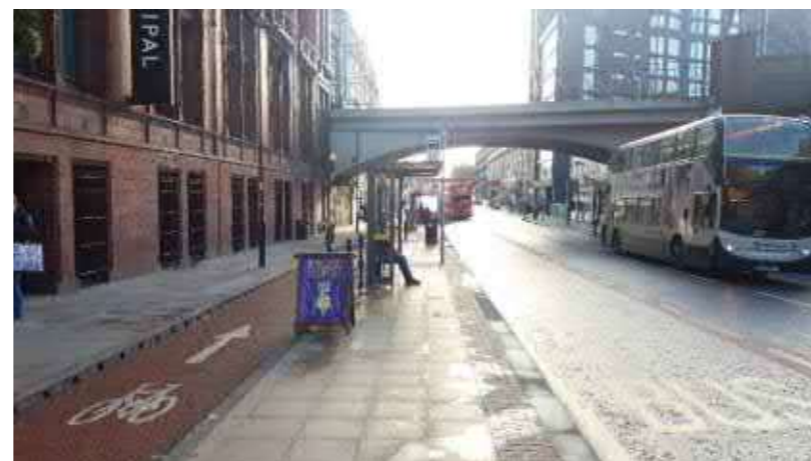
Figure 3.8. Segregated cycleway (carriageway height)
