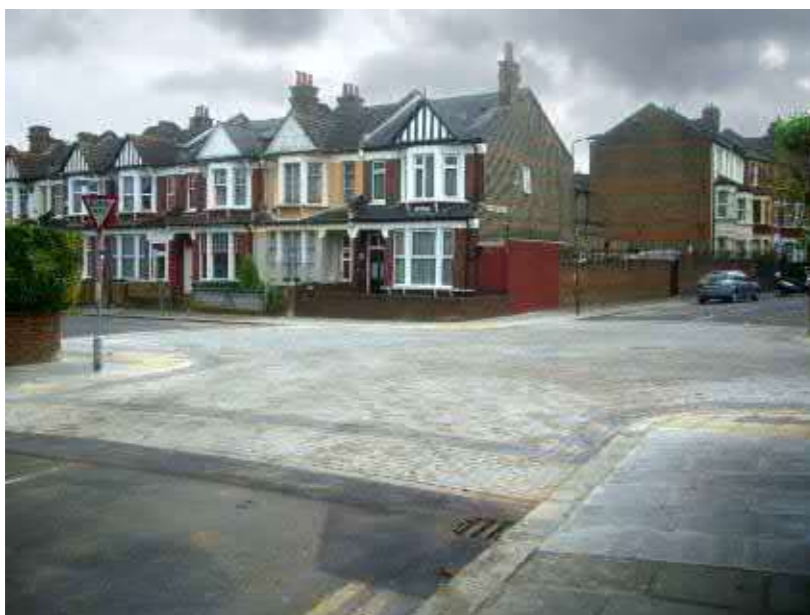
Figure 4.9. Raised table junction
